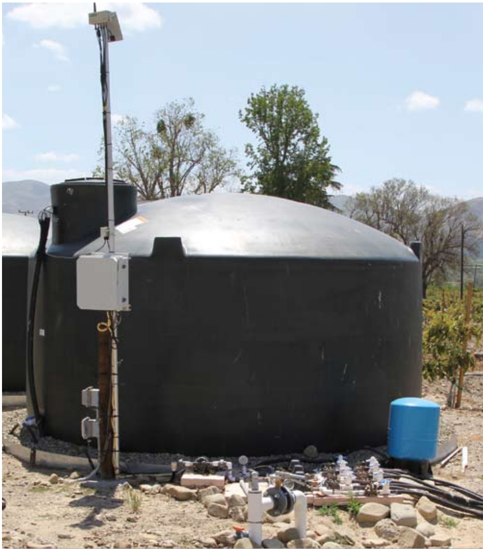
The water tank, irrigation controller, valves and flow meters used for the soil moisture sensor trial planting.
