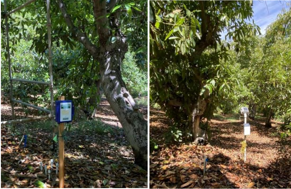
Fig. 2. Three different types of soil moisture sensors installed in multiple depths to monitor soil water and salinity status over the season on a continuous basis (avocado orchard in Irvine).
