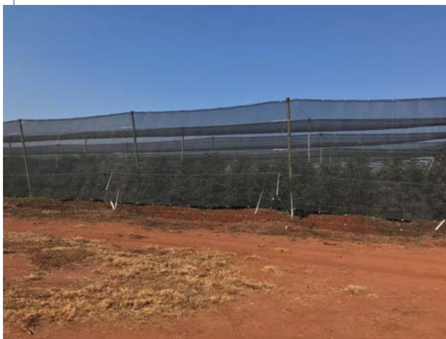
A large screen structure constructed in a grove in Soekmekaar, Limpopo Province, South Africa to protect trees from hail and wind damage.
