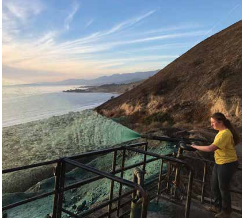
After the Thomas Fire, the Sheaffers applied hydromulch on the slopes above the town of La Conchita before the heavy rains came to prevent soil erosion.
