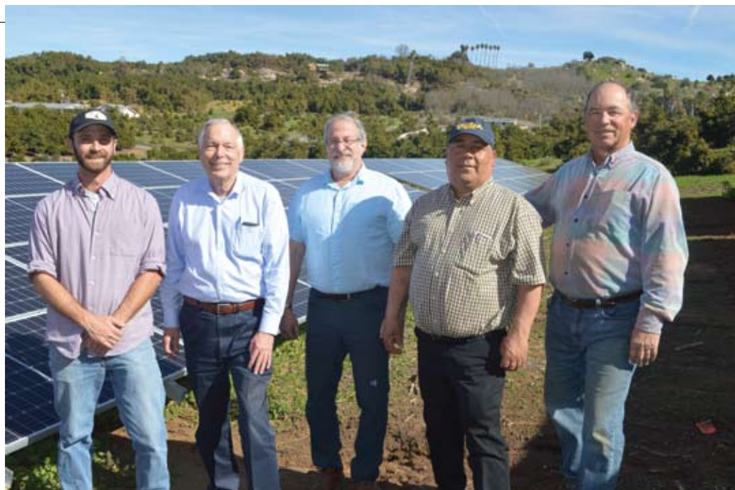
Connor McClelland, Phil Henry, Norm Kachuck, Serafin Michel and Larry Slominski pose in front of the new solar installation at ACA ranches.
